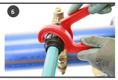
Using C ring wrenches fully tighten the nuts onto the body of the fitting
