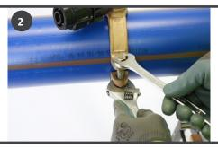
Equally tighten the nuts on both sides of the tapping tee
