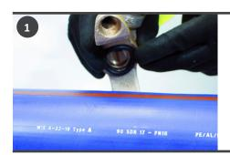
Place the O-ring into the recess of the tapping tee base and place the fitting onto the main
