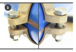
Ensure the distances between the 'lugs' are identical and parallel on both sides
