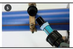
Slide the grip ring so it is flush with the pipe end and push the pipe fully into the tapping tee outlet
