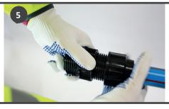
Hand tighten the nut onto the body of the fitting
