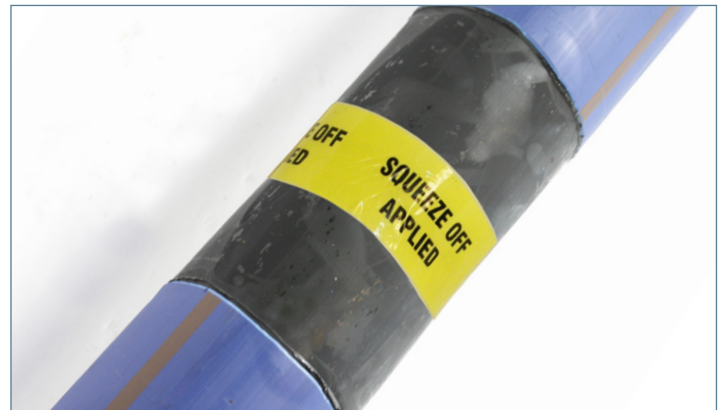
Fig. 10 'Squeeze off applied' tape on pipe following squeeze off and re-rounding
